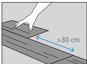
5. For the second and each subsequent row, take a new panel and decide how large the panel should be (or use a piece that is left over from one of the previous rows). For boards, make sure that the joint of the short side is at least 30 cm from the joint of the short side of the previous row; and at least 20 cm for tiles.
